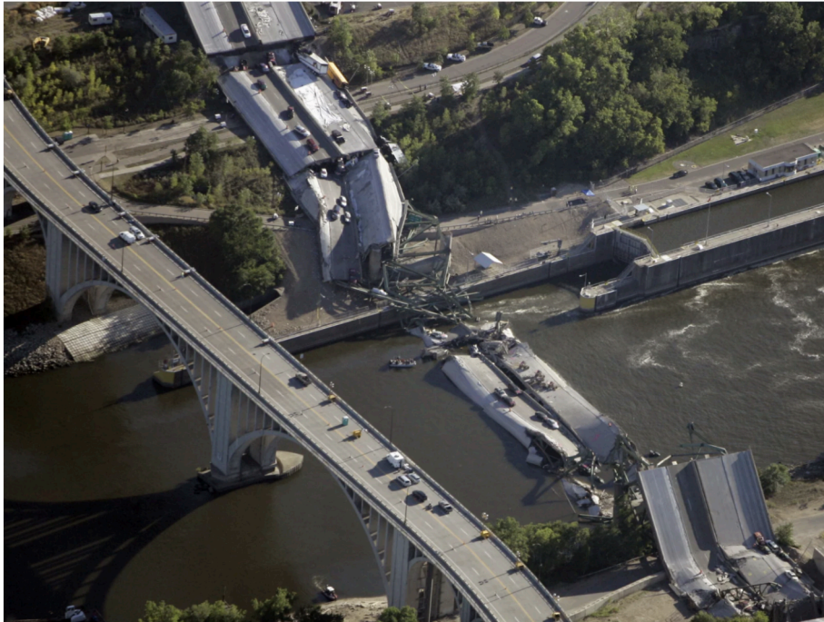
The collapsed 35W bridge in Minneapolis seen on August 2, 2007. Morry Gash/AP
